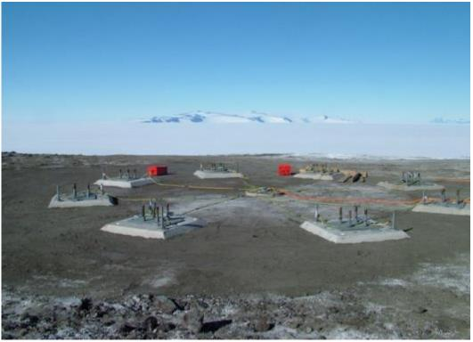
Figure 53: Pre-cast concrete foundation footings backfilled so only the top is visible.
