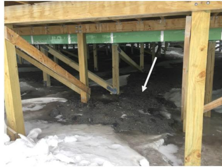
Visible ACM fragments under the Administration building
