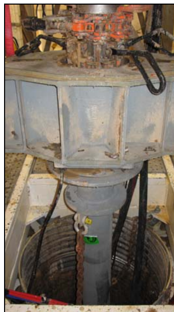
Figure 5. Borehole – top of sea riser
